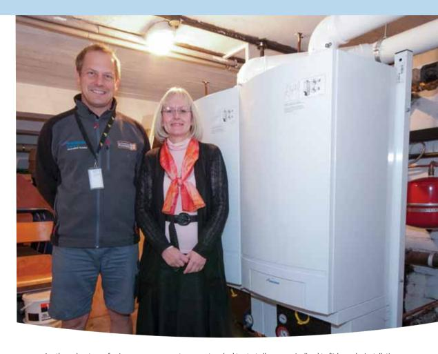
Another advantage of using a GB162 boiler is that it is incredibly quiet when in operation due to its low resistance and high quality insulation, making it ideal for inclusion in a church as it won't disturb the service.
