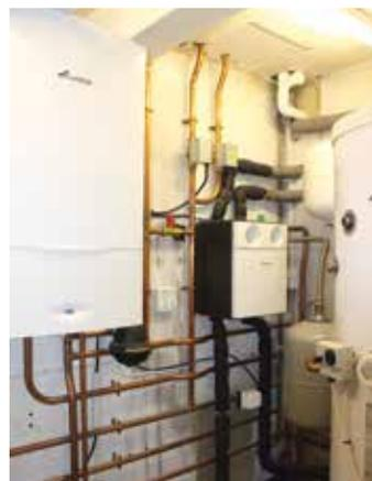
I suggested creating a zonal heating system to reduce bills and stop heating unwanted areas. The design of the previous heating system meant it was easy to interrupt the pipework and install modernised valves so rooms could be independently zoned.
