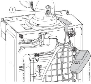
Fig. 69 Combustion test
