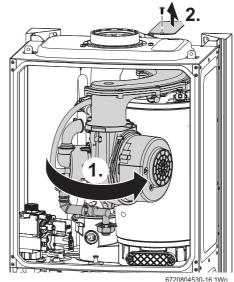
Fig. 64 Rotate air/gas manifold
